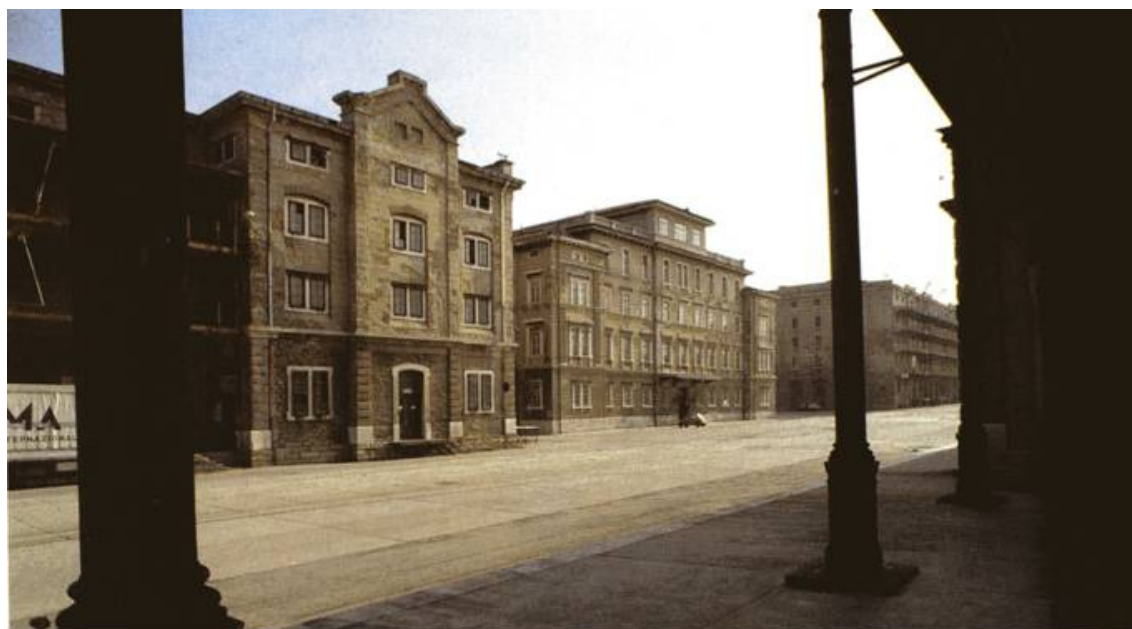
Figure 2: Snapshot of buildings of Trieste Old Port.
